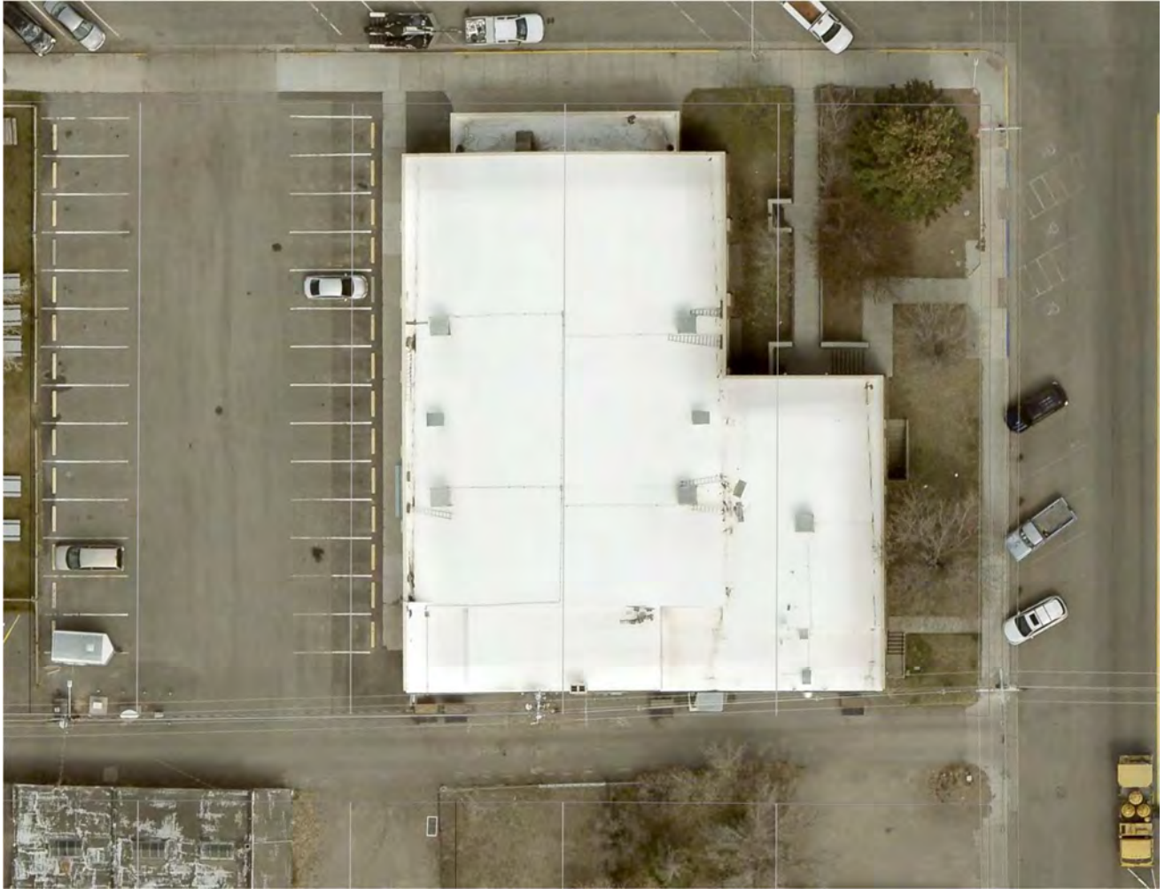
Aerial Photo of Cody Auditorium Roof.
