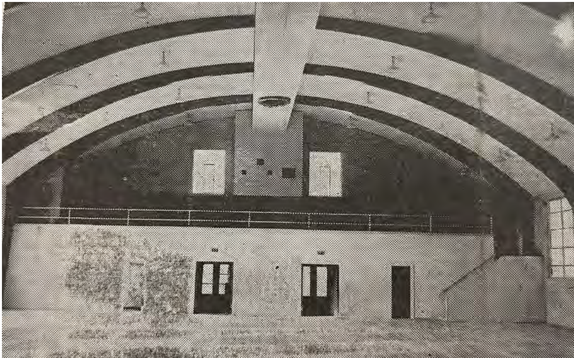
Photo Looking North from the Auditorium Towards the Lobby. Notice the Seating Area Above.
