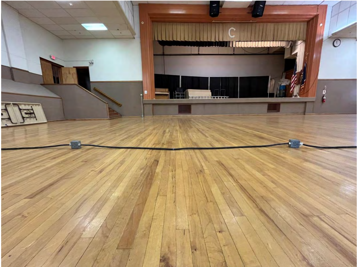
Photo of cable and floor boxes extended across auditorium floor.
