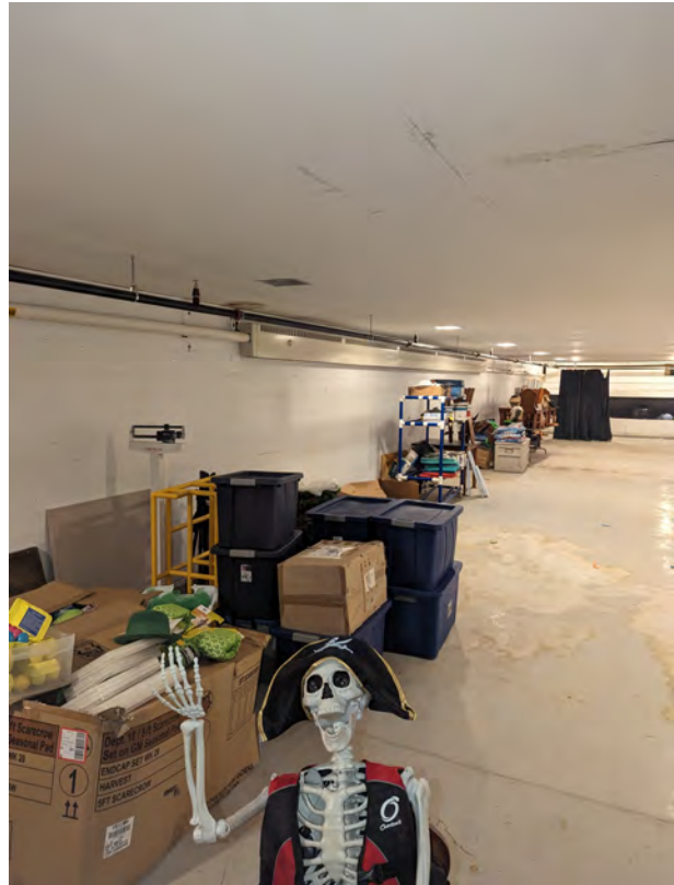
View of slab on grade (Item S3).
