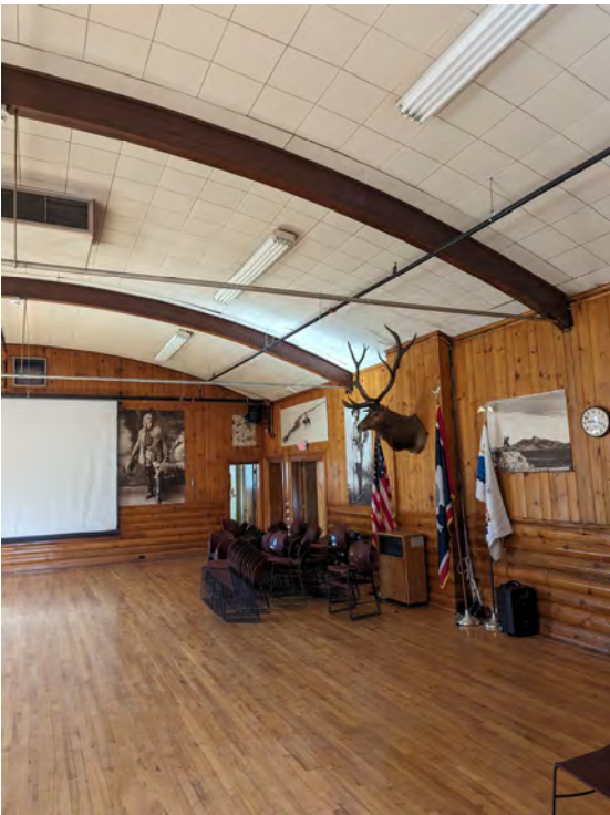
View of curved glu-lam beams (Item S4).
