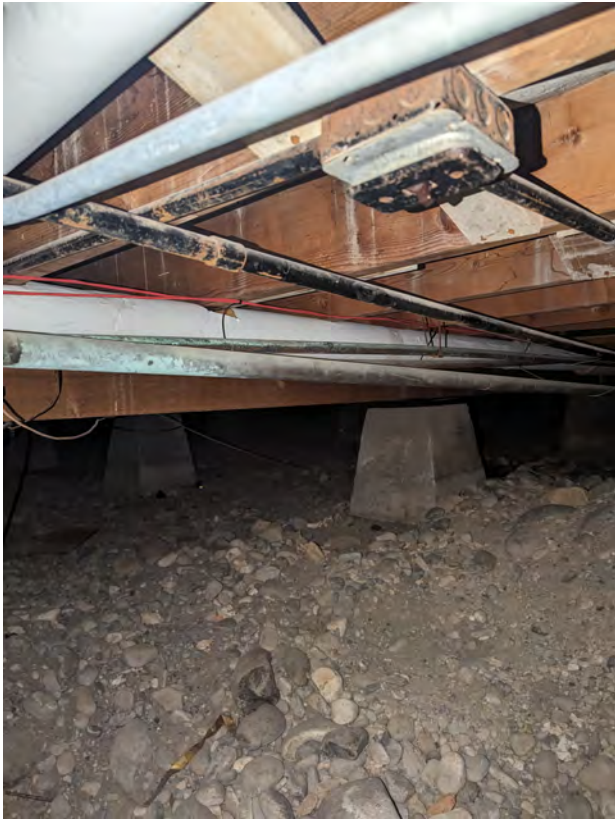
View of floor framing on footers (Item S5).
