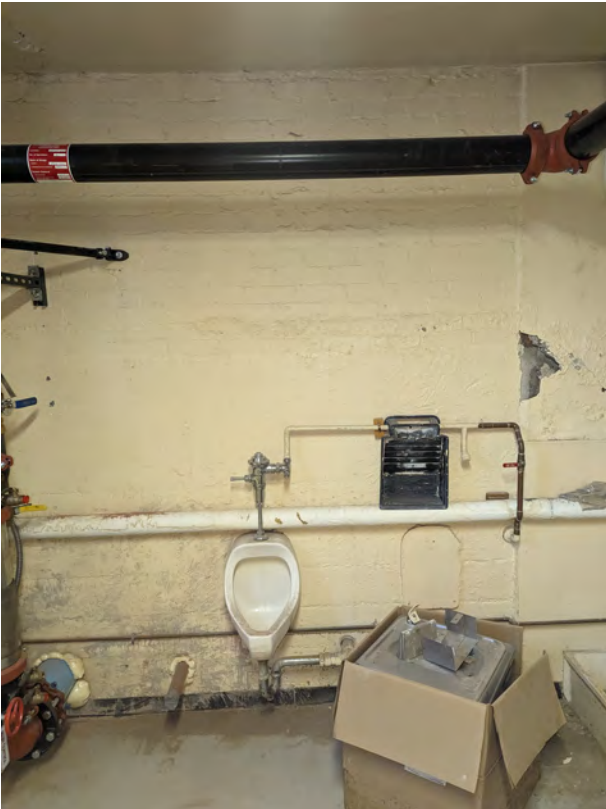
View of perimeter foundation walls (Items S1 & S2).
