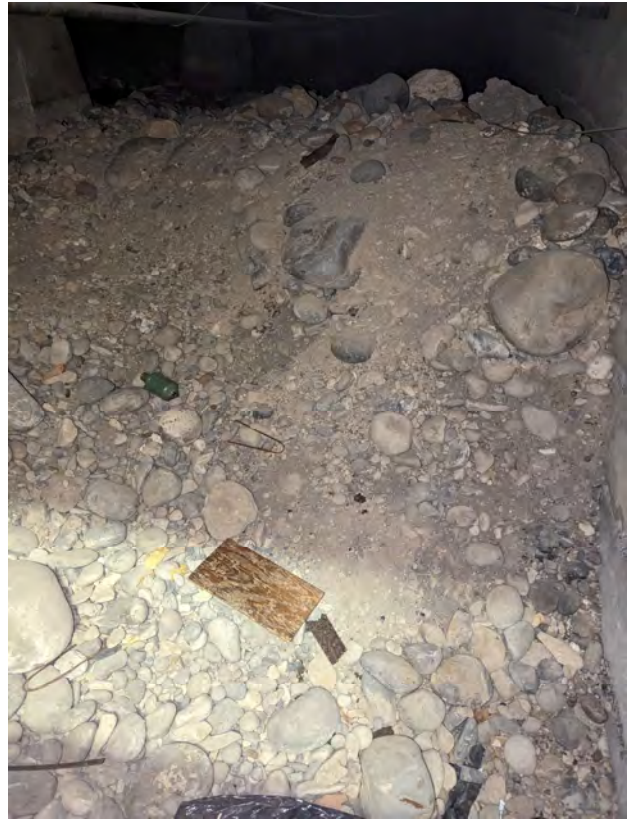
View existing Cody cobbles soils (Item S5).
