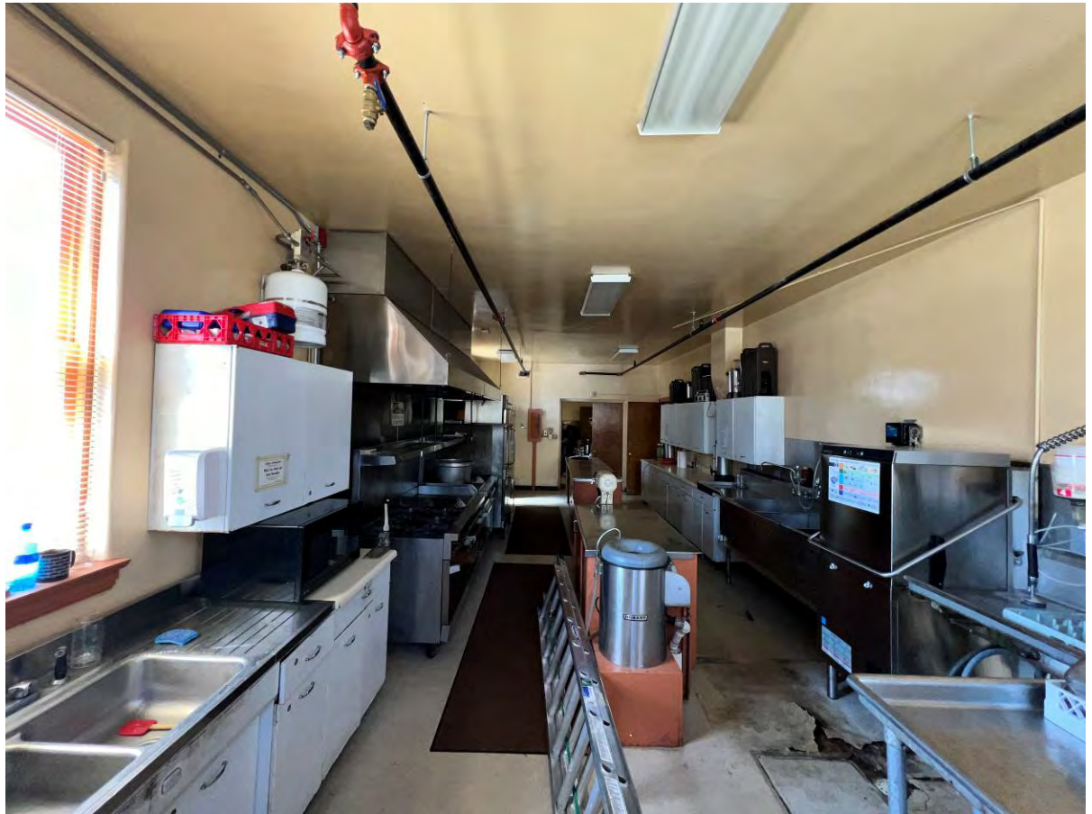
View of kitchen
