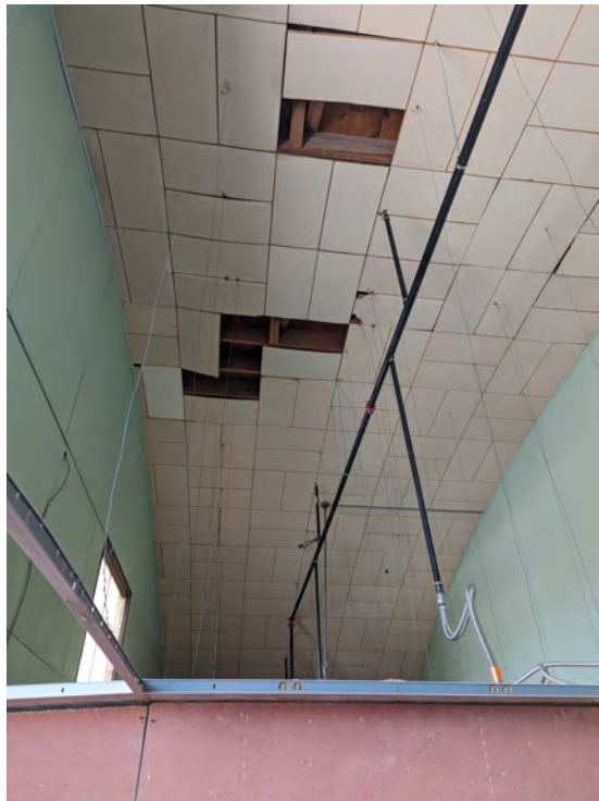
View of roof framing and decking (Item S4).
