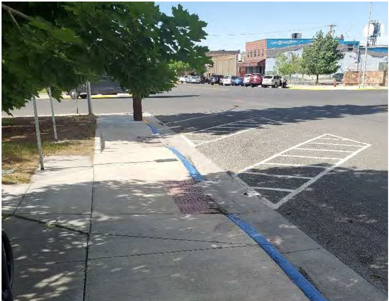
Photo of ADA parking and ramps.
