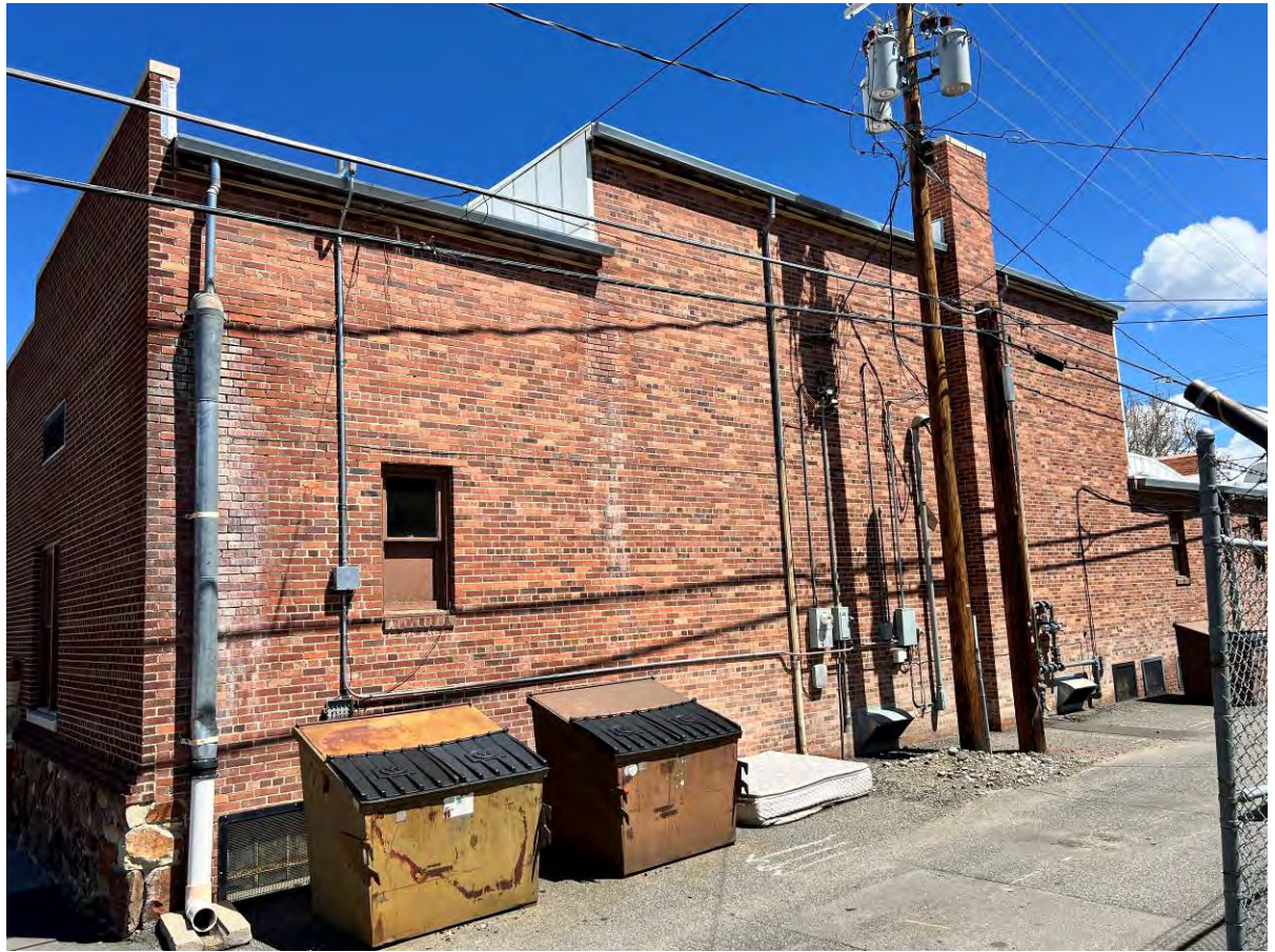
Roof Gutter and downspout
