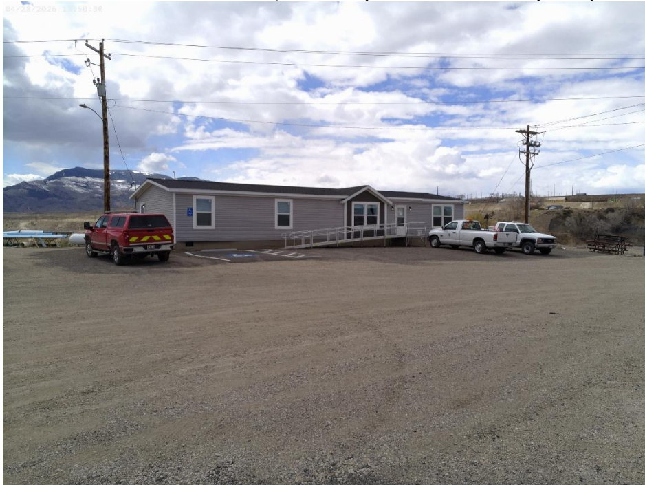
Photo of the office structure, currently in use at the City Shop at 119 19 th Street.
