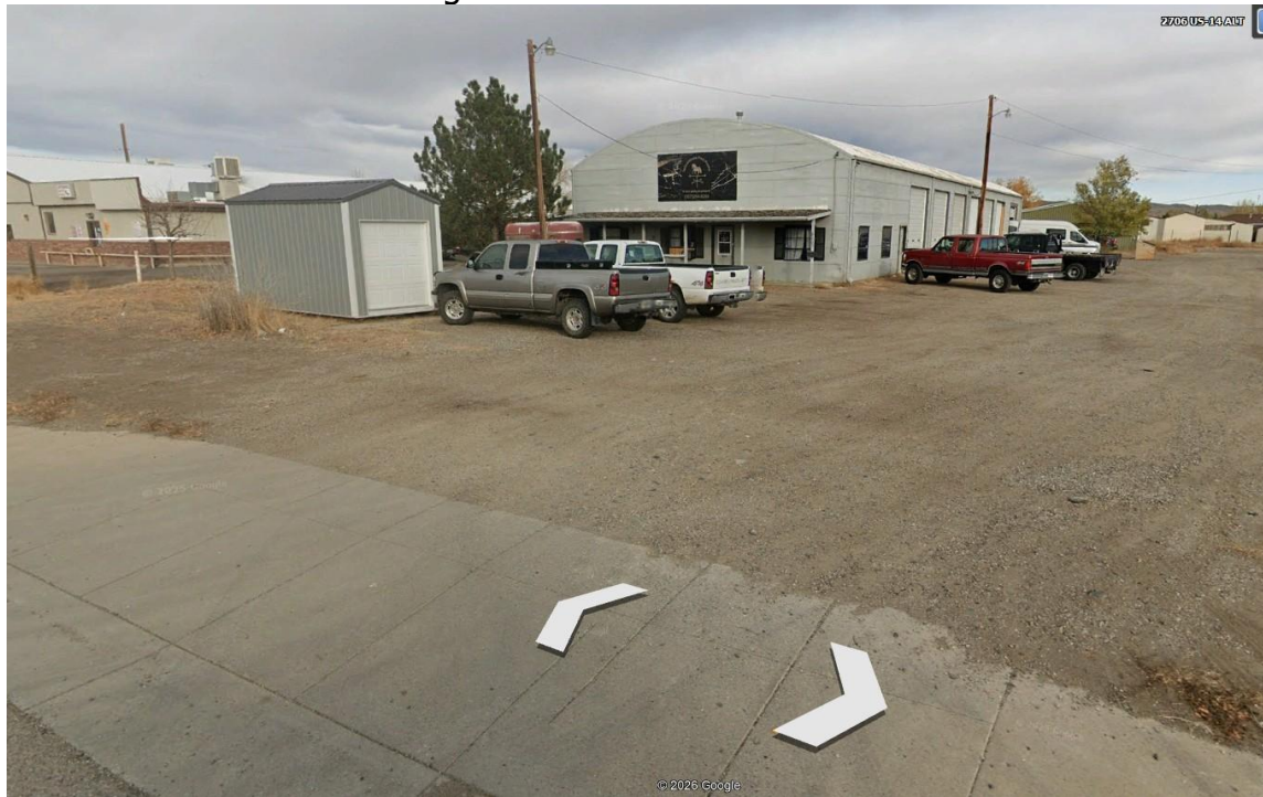
Structure located at 2707 Big Horn Avenue.
