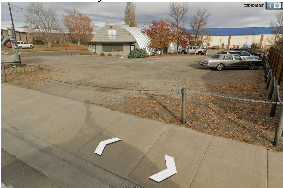
Structure located at 1901 Big Horn Avenue.
