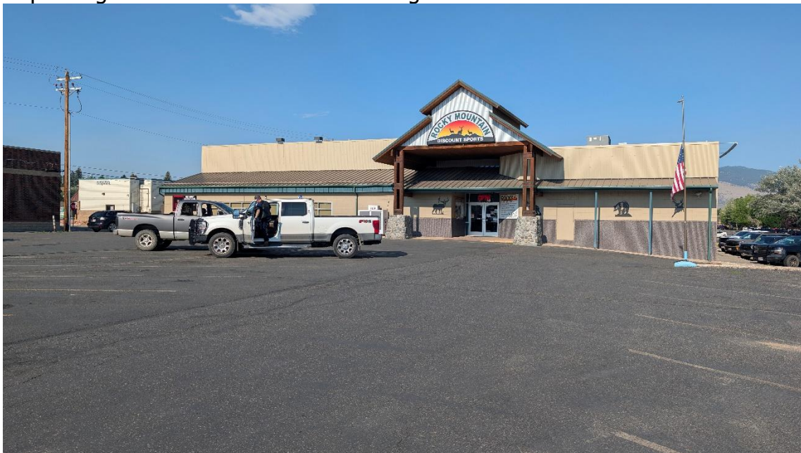
Photo of the entrance to the building, showing the north tenant space (right) Rocky Mountain Discount Sports. The left side of the building is the south tenant space requesting allowance for attached wall signs:
